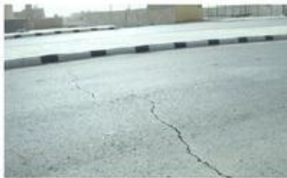
Transverse Crack
