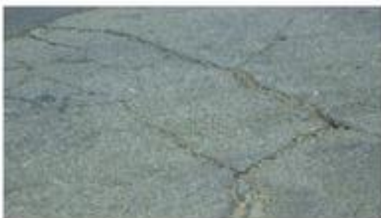
Block Crack
